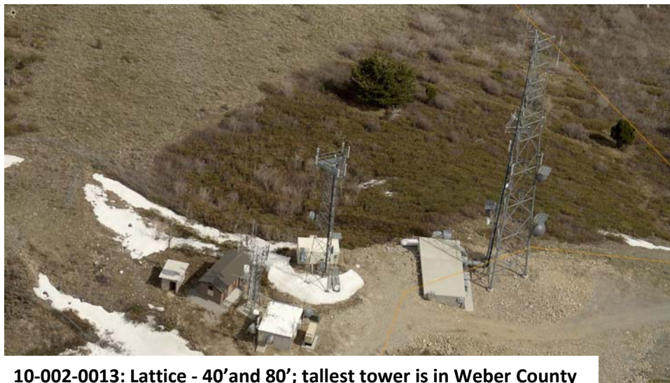
10-002-0013: Lattice - 40' and 80'; tallest tower is in Weber County
